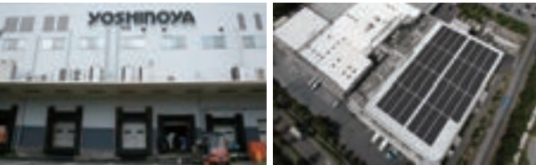
Yoshinoya Tokyo factory introduces solar power generation
