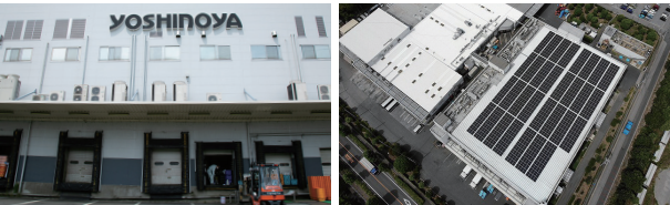
Yoshinoya Tokyo factory introduces solar power generation
