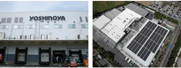
Yoshinoya Tokyo factory introduces solar power generation
